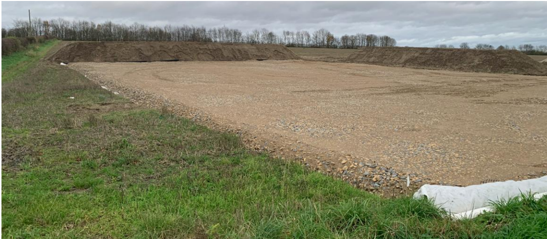
Insert 21: Newly-laid Construction Compound (Elsham-Lincoln Pipeline)
