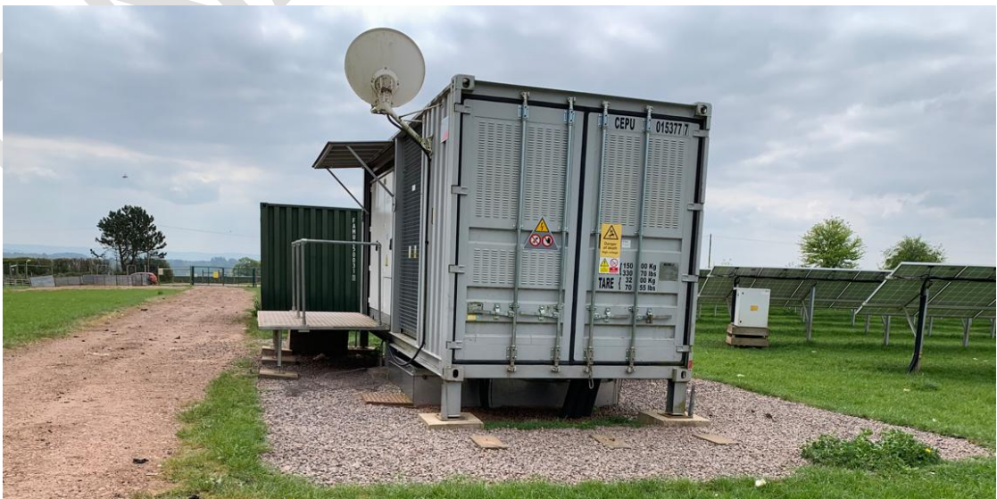
Insert 24: Typical Inverter Containers
