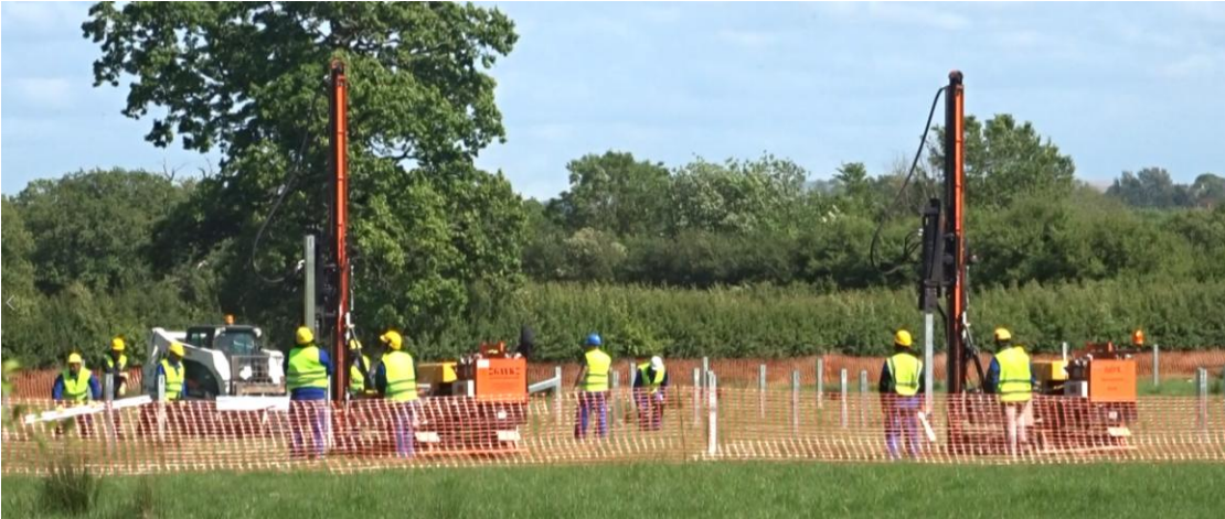
Insert 5: Team Installing Panels
