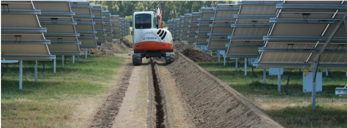
Insert 19: Cable Trenching, Central Row
