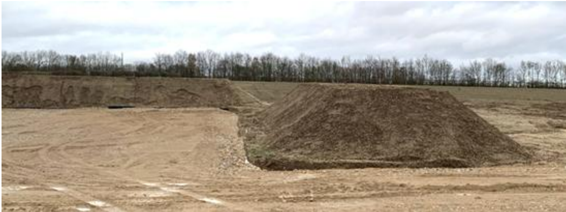
Insert 23: Example Topsoil Storage Bund
