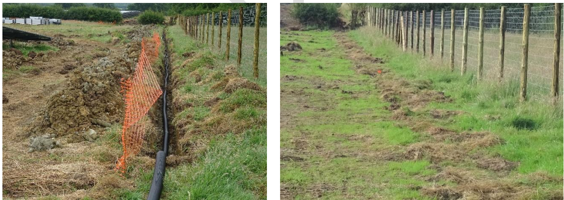
Inserts 17 and 18: Example of Cabling Being Installed (Purton)
