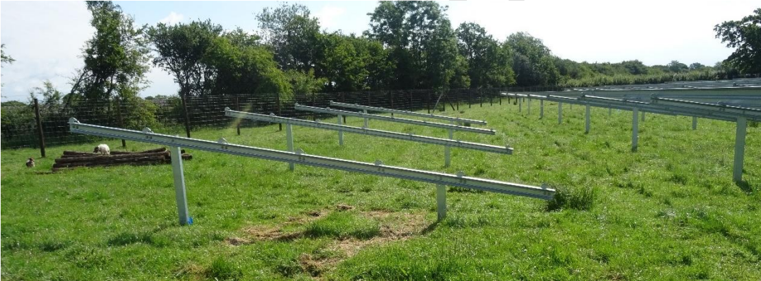
Insert 7: Legs being Installed (this at Tiln Farm, Retford, January 2023)
